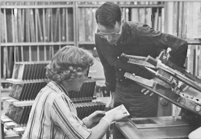
Circuits are printed by silk screen process on boards with great skill and precision by Elfriede Gmelin.
